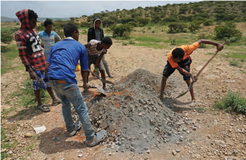
Figure 9.3 Concrete mixing training.
