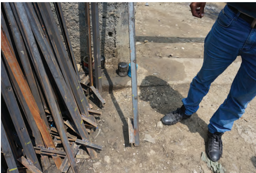
Figure 9.10 L-type metal column preassembled by cutting and welding.
