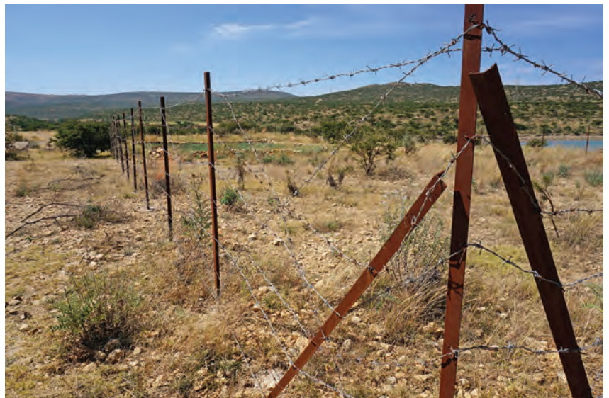
Figure 9.12 L-type metal fence with barbed wire surrounding the reclaimed farmland.
